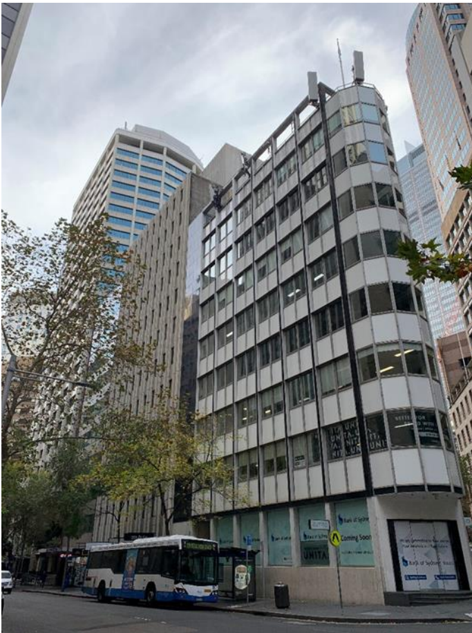
Figure 19 – Liverpool & London & Globe building, viewed facing north-east along Pitt Street.
