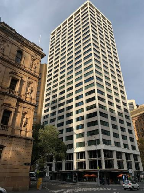
Figure 15 – Building at 56 Pitt Street, viewed facing south-west on Bridge Street.
